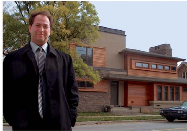
Architect Richard Librach designed this controversial modern home at Ledbury and Fairlawn
